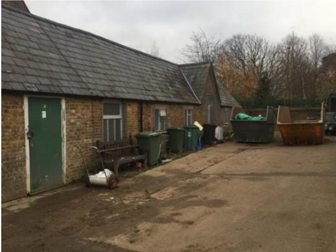
Figure 2: Existing Depot courtyard
