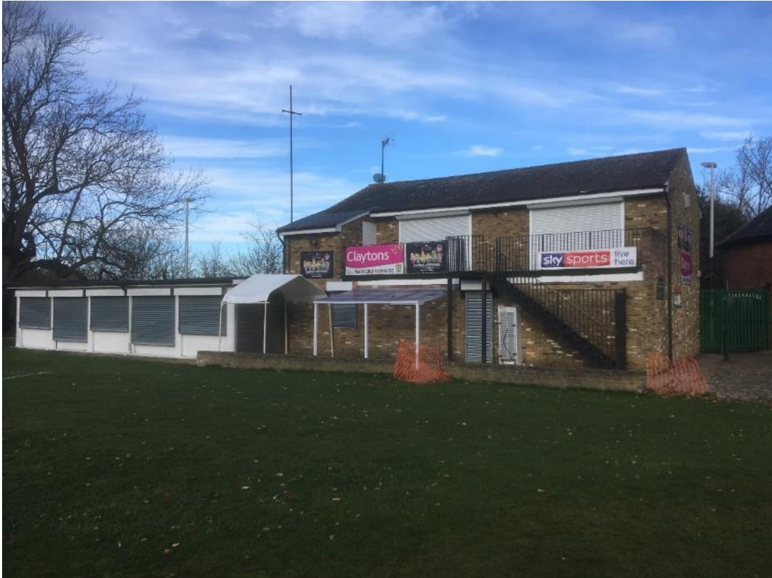
Figure 3: Existing Cricket Pavilion
