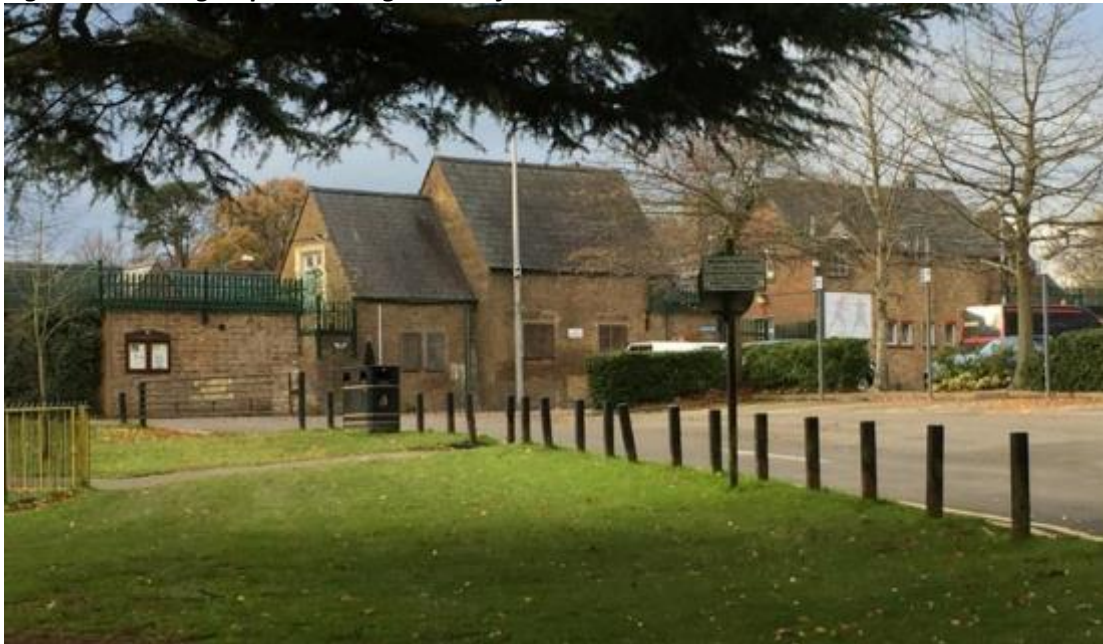
Figure 1: Existing Depot building viewed from
